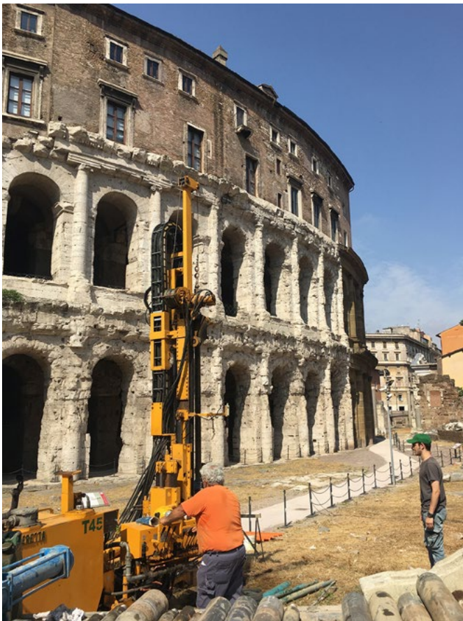
Drilling cores outside the Theater of Marcellus, Rome.
