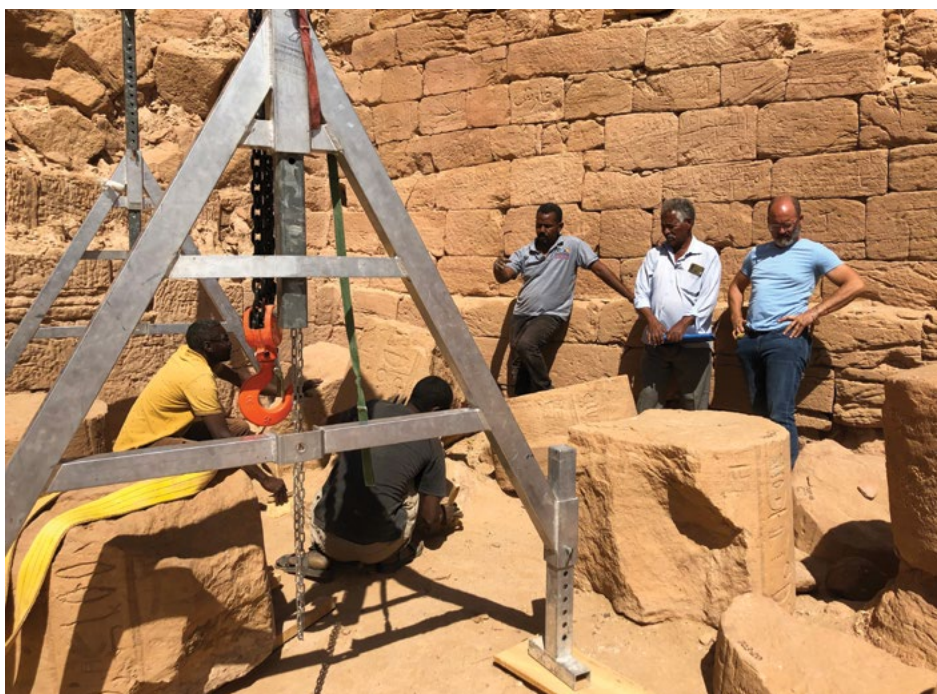
Figure 1. From left to right, conservator Elmontaser Dafalla with an assistant, conservation builder Sefian Mutwakil, archaeologist El-Hassan Ahmed Mohammed, and conservation architect David Flory discuss resetting fallen column drums in Temple B700—a temple dedicated to the Nubian god Osiris-Dedwen—at Jebel Barkal. Photo by Suzanne Davis.
