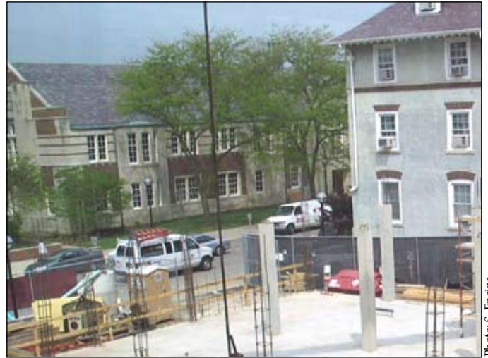
2. View of first floor after the floor and columns have been poured.
