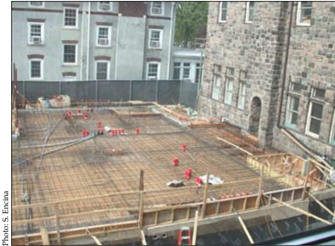
1. View of first floor before the floor is poured.
