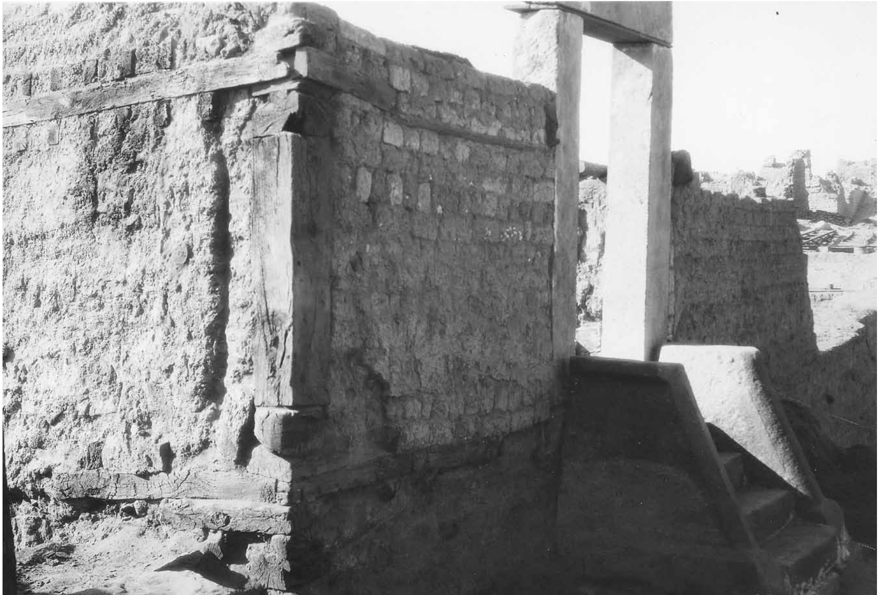
Fig. 3. "House of the Banker" (C401/B501). The impressive stone entrance, unusual among the mud-brick houses of Karanis, is probably a sign of the proprietor's wealth. In the underground rooms of this house some 26,000 coins were found stored in jars and cloth bags (Kelsey Museum Archives, 5.4247).
