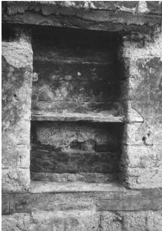
Fig. 42. Cupboard niche in the wall of House C57; within the niche a wooden shelf is well preserved (Kelsey Museum Archives, 5.2800).
