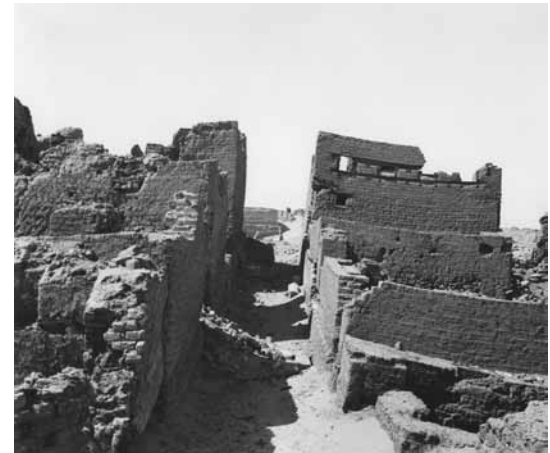
Fig. 34. Walls of mud brick laid in concave beds appear to sag in this view along Street C552 (Kelsey Museum Archives, 828).
