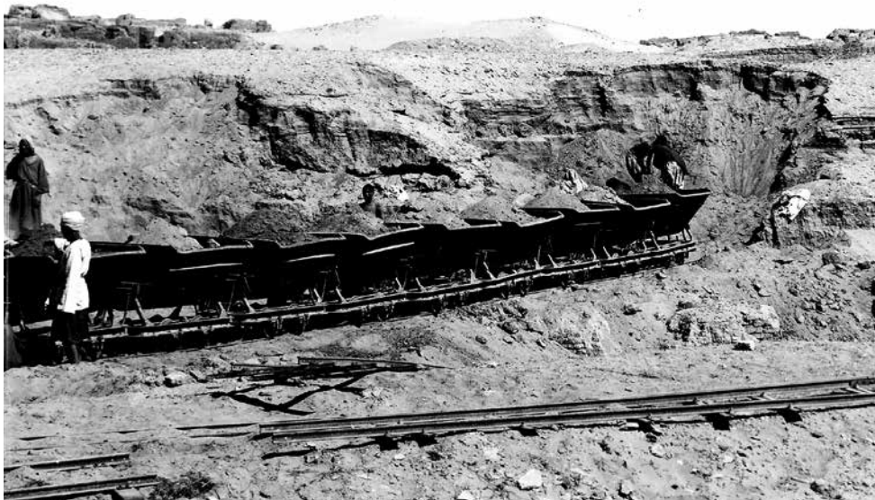
Fig. 5. Building a railway for the removal of sebakh from the site (Kelsey Museum neg. no. 5.2466).
