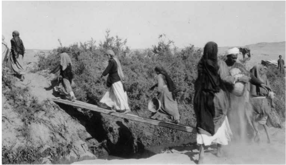
Fig. 6. Scene at the canal when the south bank broke: repair work, 24 December 1925 (Kelsey Museum neg. no. 655).
