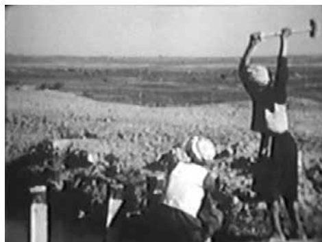
Fig. 10. Workers repairing a canal (Karanis motion pictures, reel Vb).
